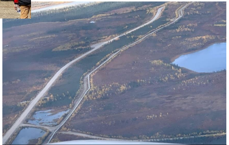
Aerial view of Pipeline and Yukon River
